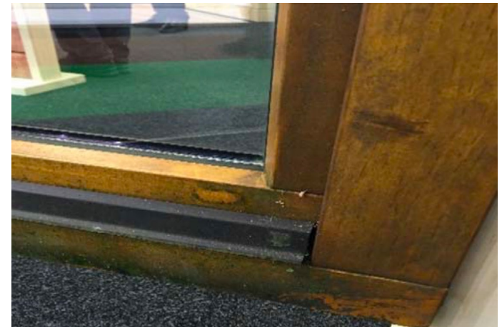
No coating degradation visible
